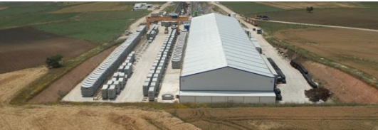
Karacabey tunnel segments
