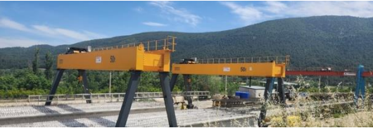
Bursa–Bilecik precast girders
