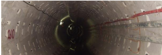
İSKİ tunnel segments
